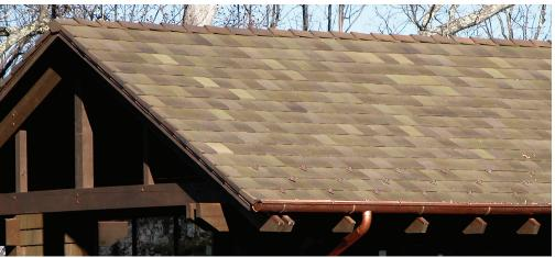
Ludowici's Lanai 14" interlocking tile has a square butt and a weathered sandblasted surface giving the aged look and character of centuries old tile. The clean, uniform look complements any architectural style. Lanai is also available in a larger 16" profile. Lanai tiles are available in all standard and custom colors, mists and blends offered by Ludowici. See the *Colors of Ludowici* brochure for more information about our extensive color program.
