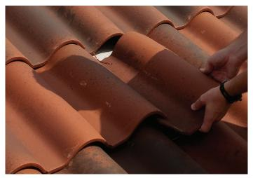
Lift the tile in the course above and slide the replacement tile into place so that the bracket engages the top of the tile below the replacement.
