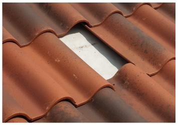
Remove broken pieces of tile and using a slate ripper, remove existing nail or screw fastener.
