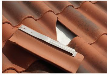
Align Quik-Tach bracket on the back of the replacement tile so that the bottom step edge is at the correct head lap. Wire the bracket to the replacement tile with copper wire.
