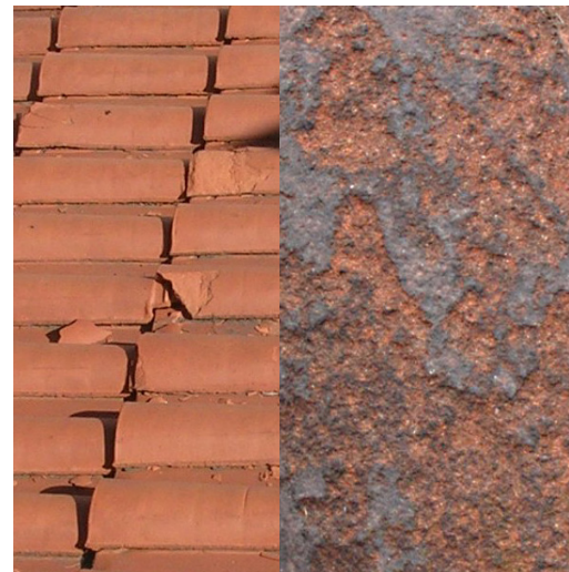
Pictured: Spalling
