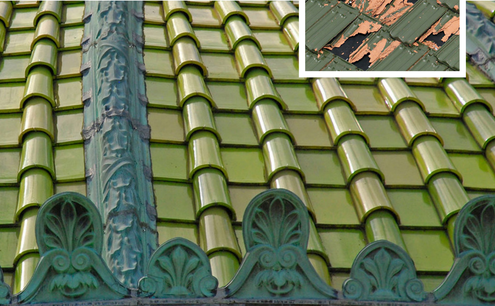
Pictured: Color permanent Ludowici roof tile (below); Imported competitor tile failure as a result of freeze/thaw issues (right)
