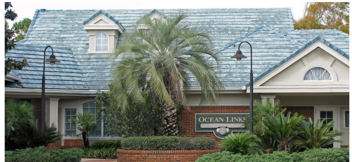
Pictured: Concrete tile failure with fading, Florida
