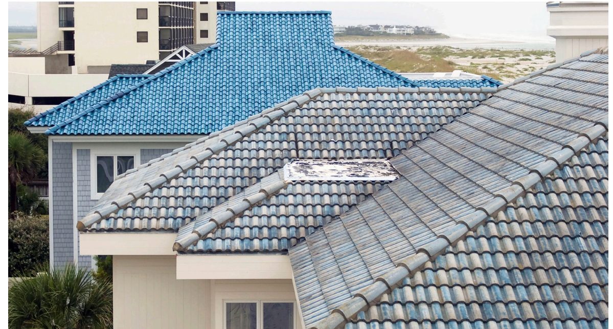
Pictured: Ludowici color permanent tile roof (back); Salt intruded and color fading concrete roof (front)
