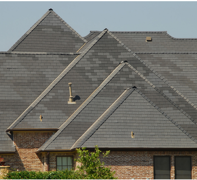
Pictured: Synthetic product discoloration and synthetic product burning (bottom right)
