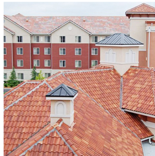
Pictured: Ludowici color permanent tile roof (front); Concrete roof with salt intrusion and fading (back)
