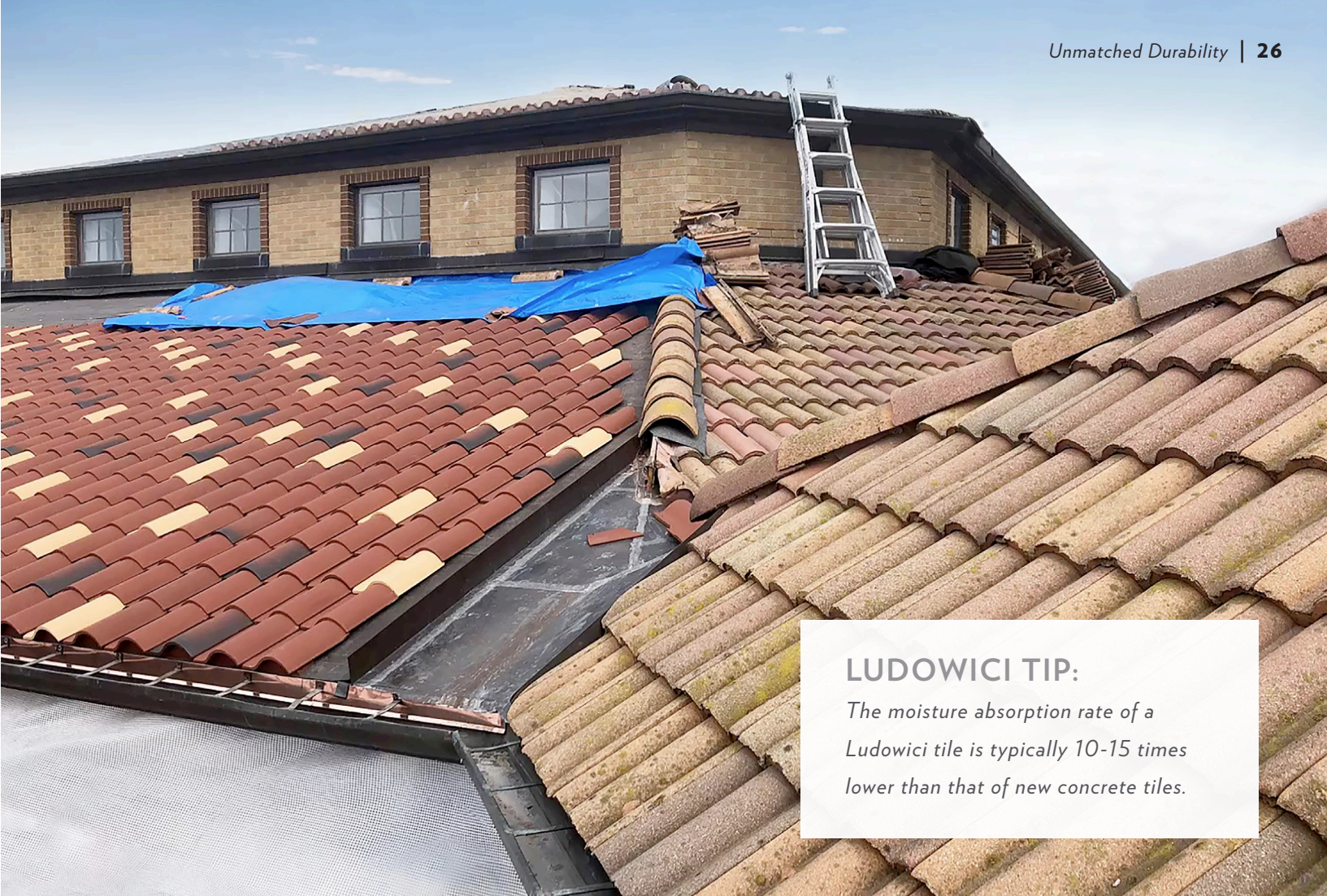
Pictured: Ludowici color permanent roof tile (left); Concrete roof with fading and mold growth (front/right)
