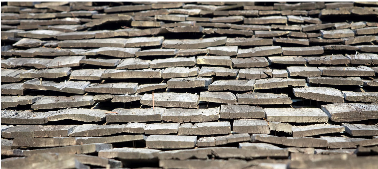
Pictured: Shake products showing warping, curling and mold growth
