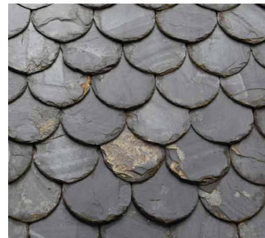
Pictured: Slate products showing delaminating and mold growth
