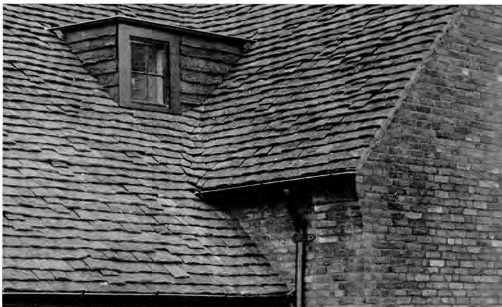
Detail of recently completed roof on which IMPERIAL Shingle Tiles were used The texture shown here is remarkably similar to that on the house at Groombridge, shown on page 12
